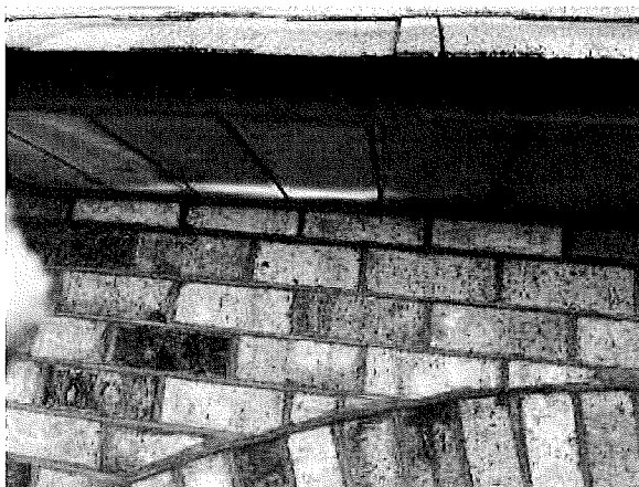
Installed soffit
