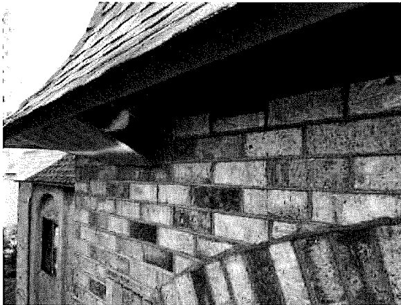
Soffit blew off due to Highwinds
